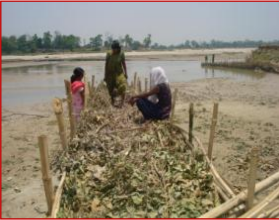
Photo 16: Filling the bamboo spur
