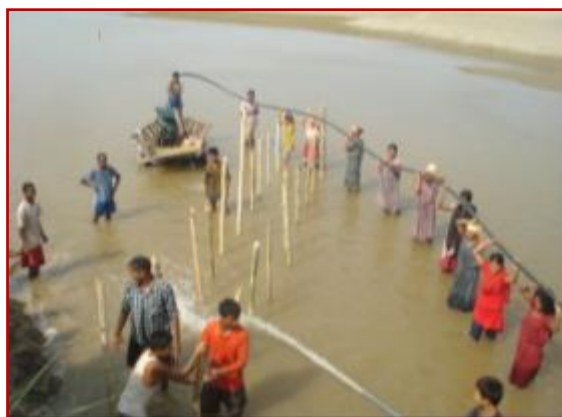
Photo 12: Placing bamboo poles for bamboo spur
