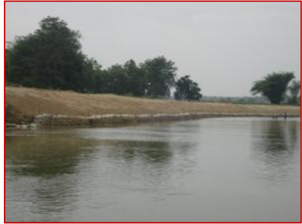
Photo 5: Bamboo crib wall and slope gradient
