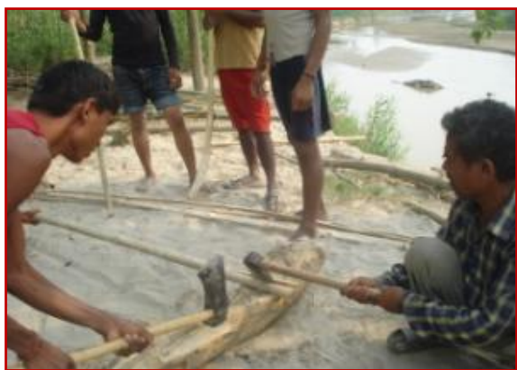
Photo 13: Splitting bamboo for crib wall
