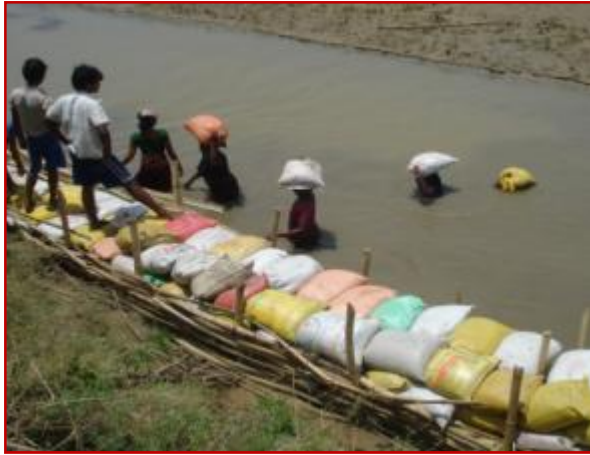
Photo 4: Filling crib wall with sand bags
