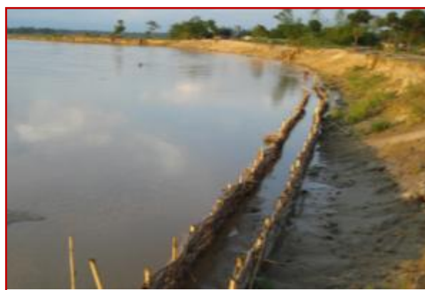
Photo 3: Bamboo crib wall
