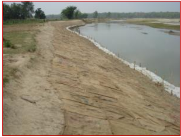
Photo 7: Jute bags on the slope
