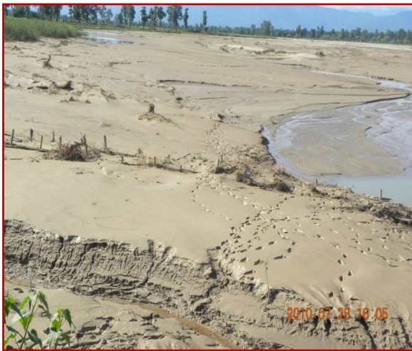
Photo 21: Sediment deposited behind bamboo spurs
