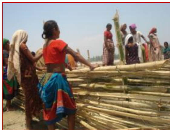
Photo 12: Placing bamboo poles for bamboo spur
