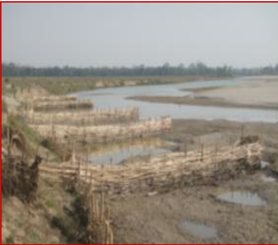
Photo 18: Bamboo wall and bamboo spurs
