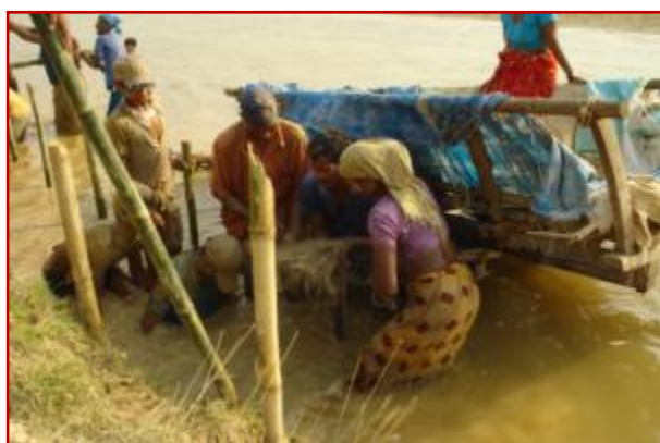
Photo 2: Placing bamboo poles
