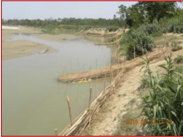
Photo 17: Bamboo wall and bamboo spur
